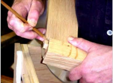
With the side fitting smoothly, I can now measure how much of the "haunch" I have to remove.
