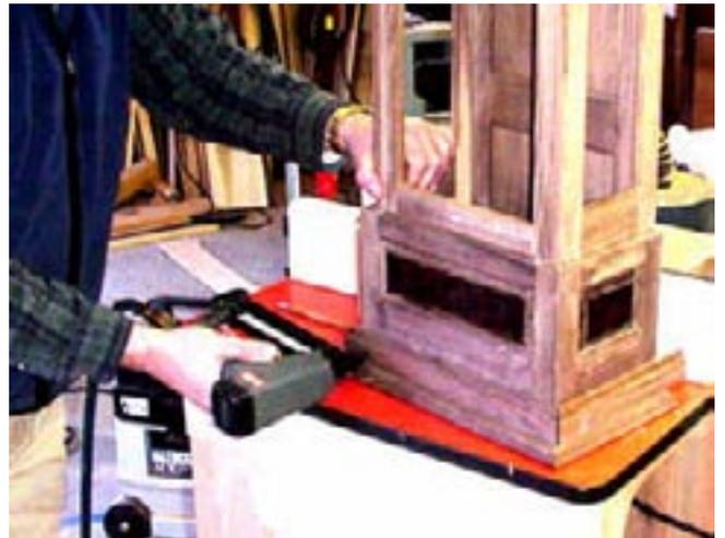
The two pieces of base molding are installed and look just fine. Now to attach the molding for just above the bottom raised panel frame. This is the one we were having trouble with yesterday.
