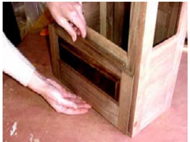
We found that there is a "best" way to add glue after dry fitting the assembly. She does not disassemble the entire frame, but instead, she removes one of the stiles at a time. With one stile off, she adds a touch of glue to where the rails will join the stiles.
