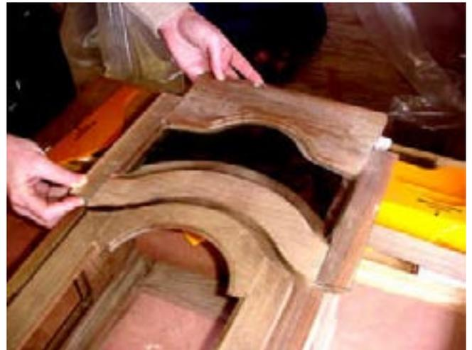
Working from the back, she attaches the template for the upper curve. As before, she uses two 5/8” sheet metal screws to temporarily secure it to the frame.
