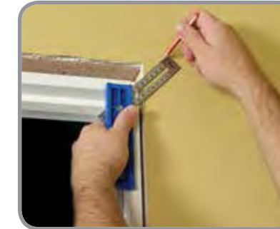
Lay Out Mitered Corners
